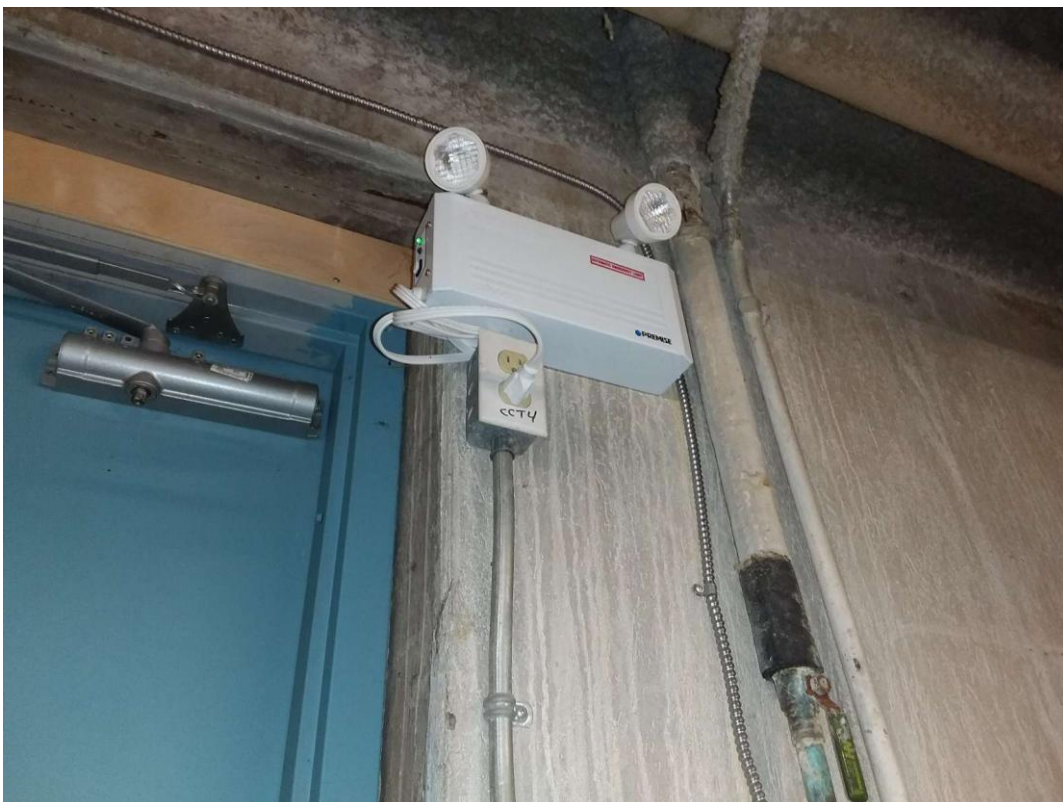
Pb Products, Presumed (V9500), BATTERIES IN EMER. LIGHTS, Furnace Room (Location #: 1)
