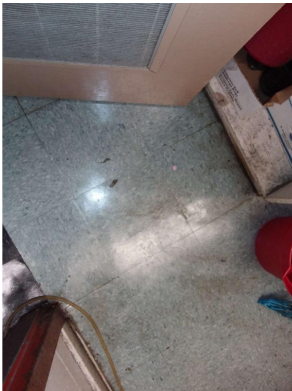
Confirmed Asbestos (detected in mastic, S0020A-C), 12" blue with blue and white flecks, Floor, Vinyl Floor Tile and Mastic, Closet (Location #: 21)
