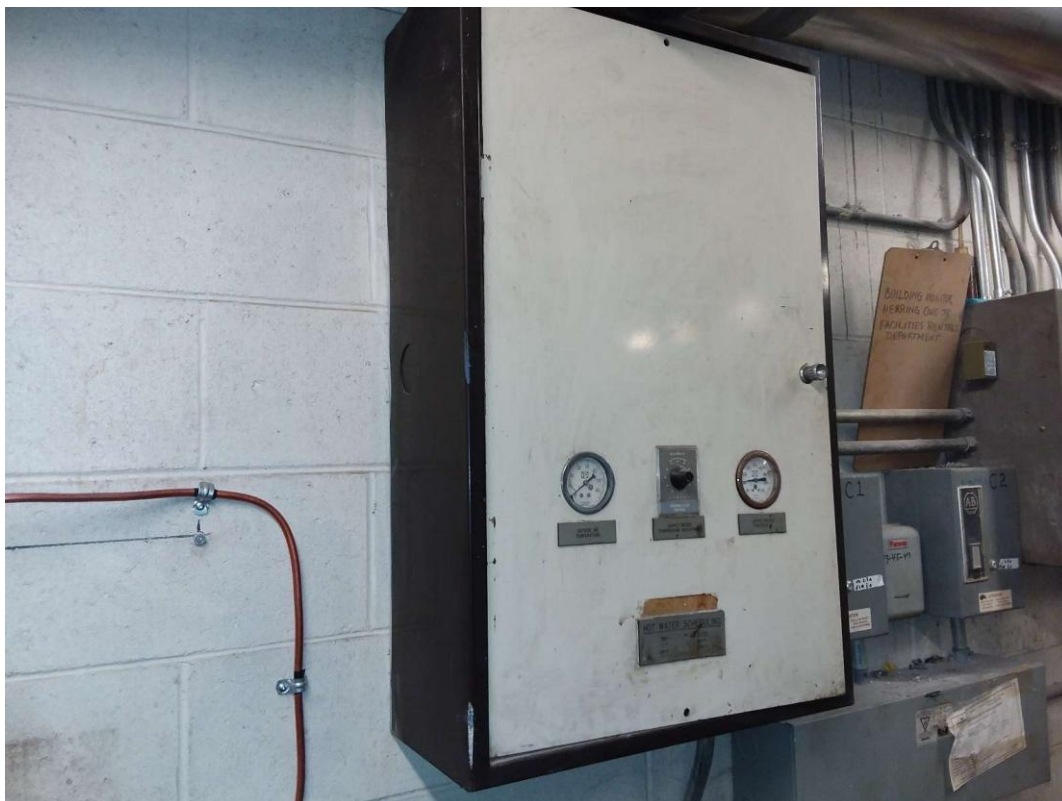
Mercury, Presumed (V9500), BOILER CONTROL, Furnace Room (Location #: 1)
