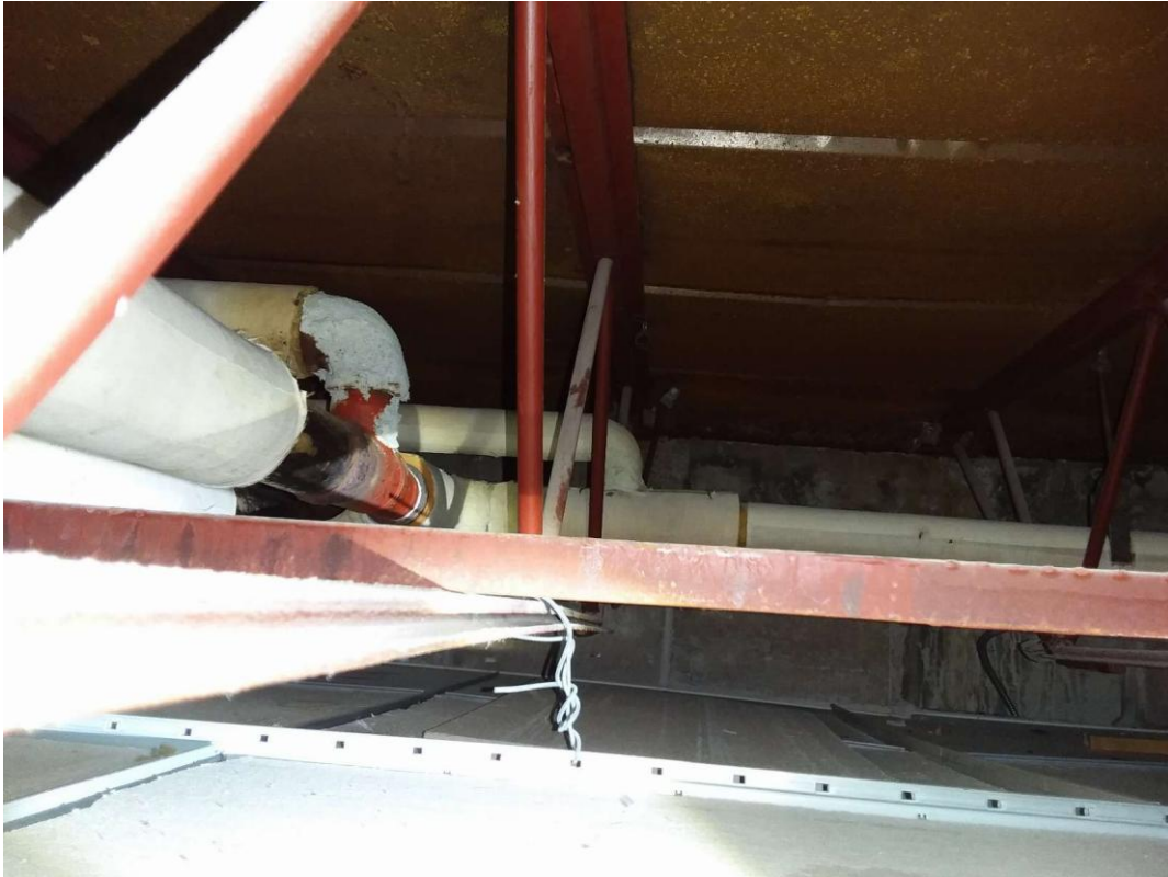
Confirmed Asbestos (S0011A-C) Piping, Parging Cement, Classroom (Location #: 6)
