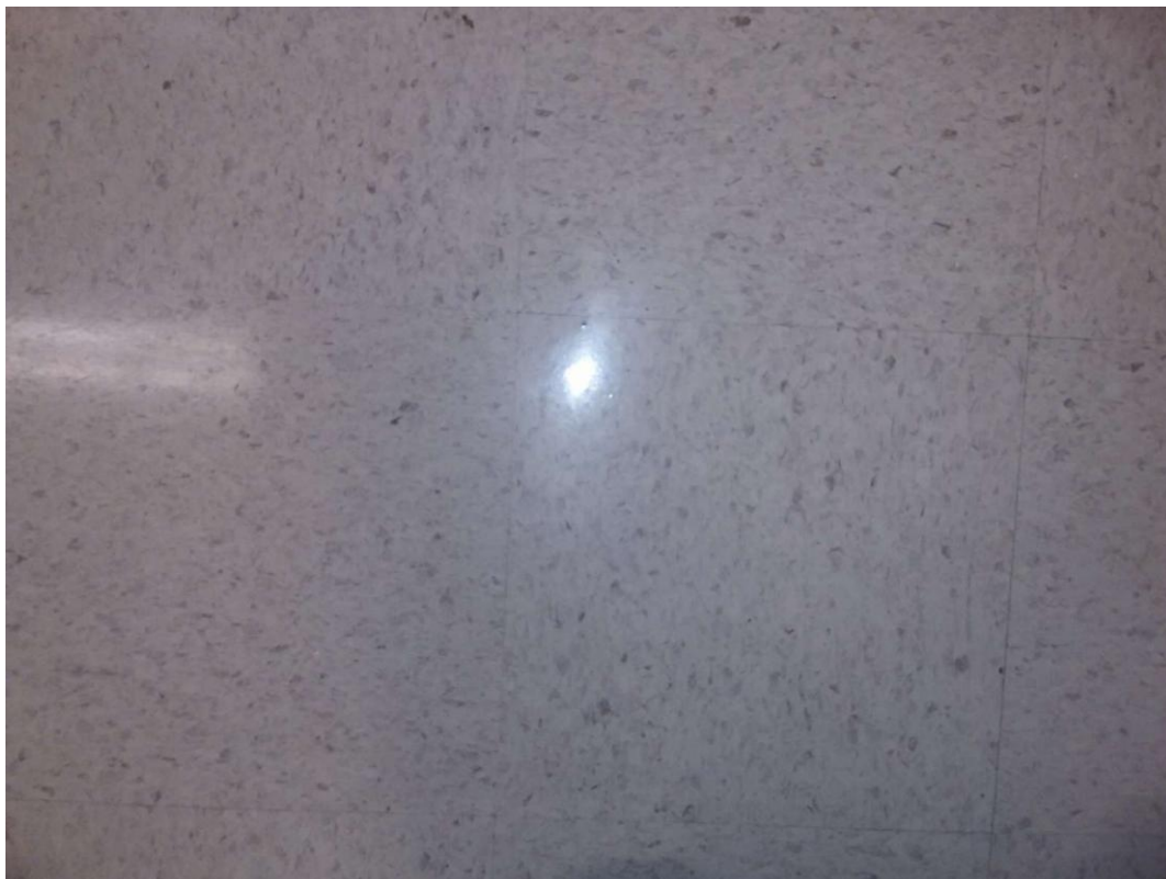
Confirmed Asbestos (detected in both tile and mastic, S0009A-C), 12" beige with light brown flecks, Floor, Vinyl Floor Tile and Mastic, Classroom (Location #: 3)
