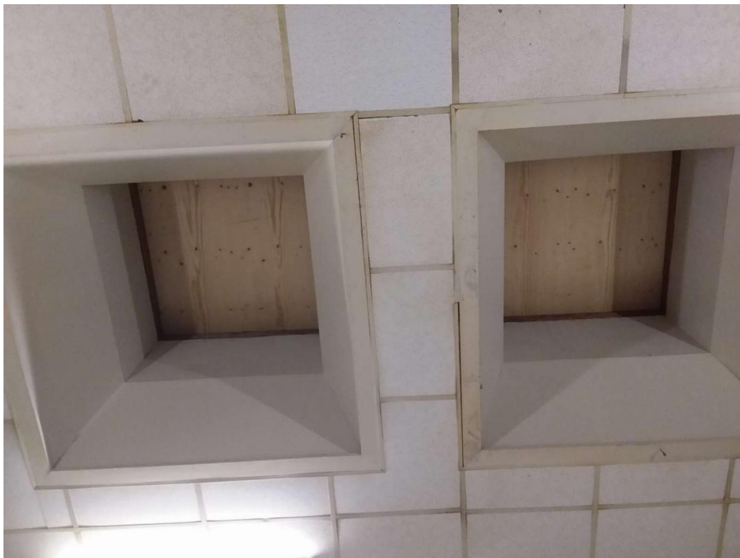
Presumed Asbestos (V9500), Other, Cement Product, Stairwell (Location #: 73) Suspect Transite tiles around sky lights
