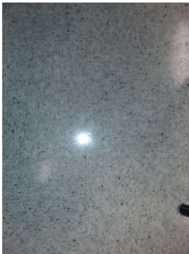
Confirmed Asbestos (detected in both tile and mastic, S0012A-C), 12" white with black flecks, Floor, Vinyl Floor Tile and Mastic, Classroom (Location #: 5)
