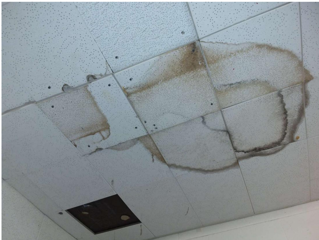
Mould, Yes (V9000), Ceiling, Ceiling tiles (glue-on), Wood Lab (Location #: 7)
