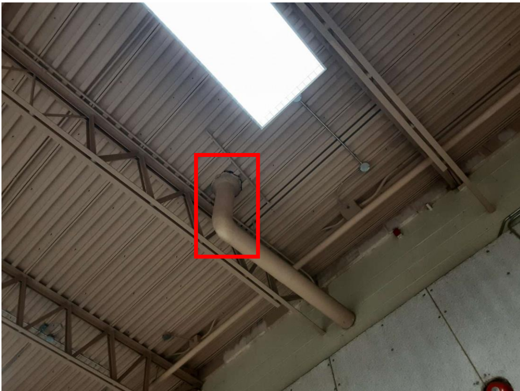
V9500 (Presumed Asbestos), Piping, Roof Hopper (Drain), Parging Cement, Gym And Stage (Location #: 52)
