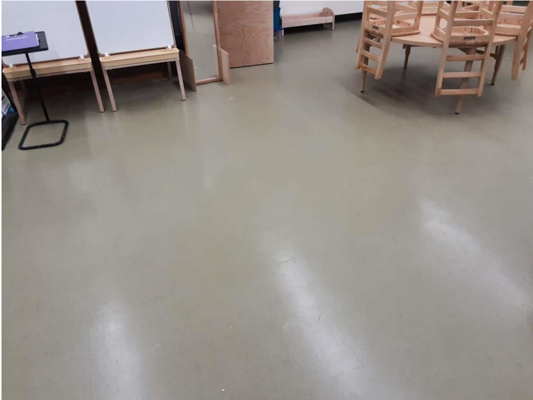
S0013B (Confirmed Asbestos), 12" forest green with faint brown streaks, Floor, All, Vinyl Floor Tile and Mastic, Classroom (Location #: 15), Asbestos detected in vinyl tile and mastic
