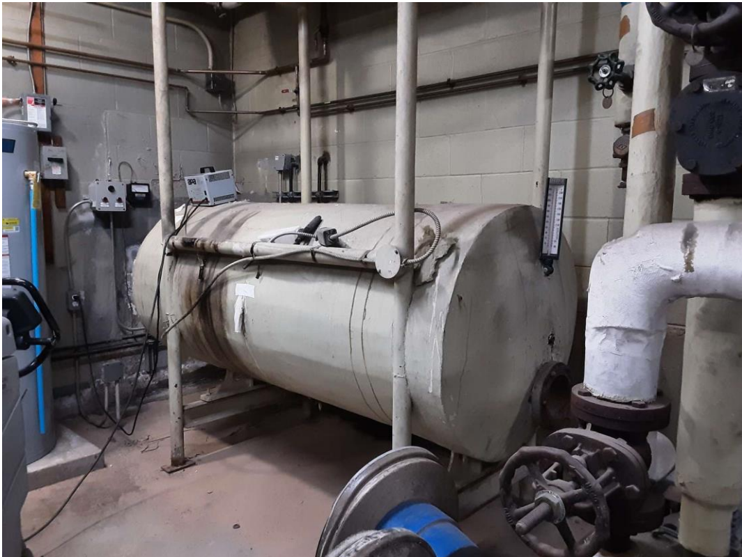
S0002C (Confirmed Asbestos), Mechanical Equipment, Heating Water Tank, Parging cement and Preformed Block, Boiler Room (Location #: 1)
