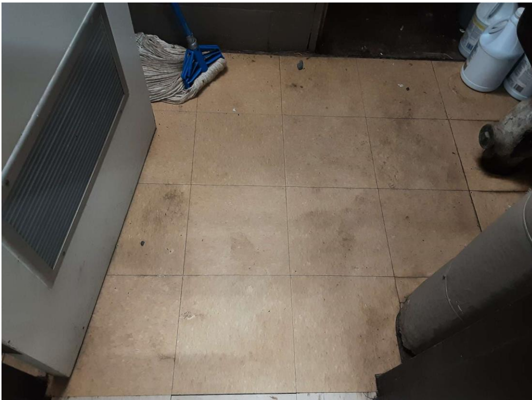
S0018A (Confirmed Asbestos), 12" light brown with flecks, Floor, All, Vinyl Floor Tile and Mastic, Janitor Closet And Pipe Chase (Location #: 26), Asbestos detected in floor mastic
