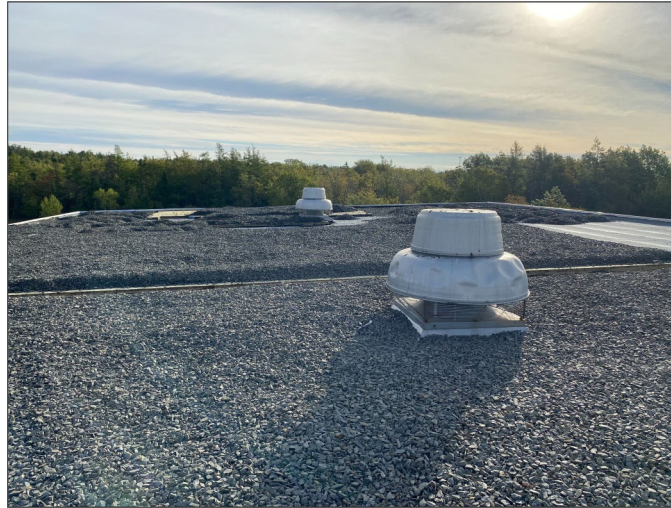
Photo 1 - General view of gymnasium roof
