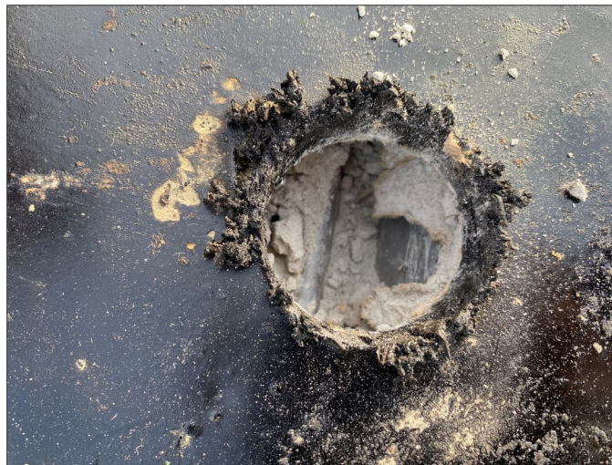
Photo 2 - S0001A-C (None detected) Roof core
