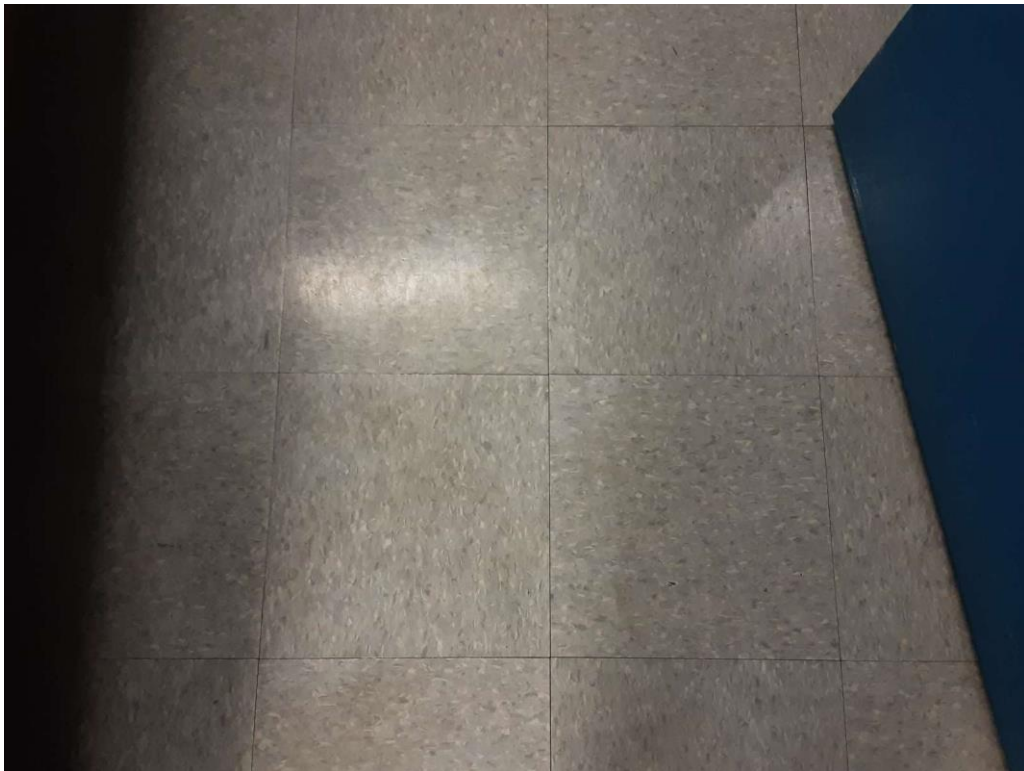
S0014A (Confirmed Asbestos), 12" medium grey with grey and white flecks, Floor, All, Vinyl Floor Tile and Mastic, Office (Location #: 14)
