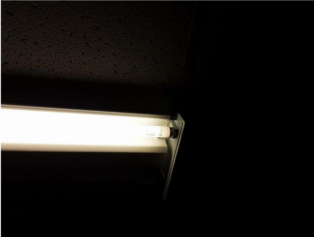
Mercury, V9000 (Yes), LIGHT FIXTURE, Caretaker Office (Location #: 25)
