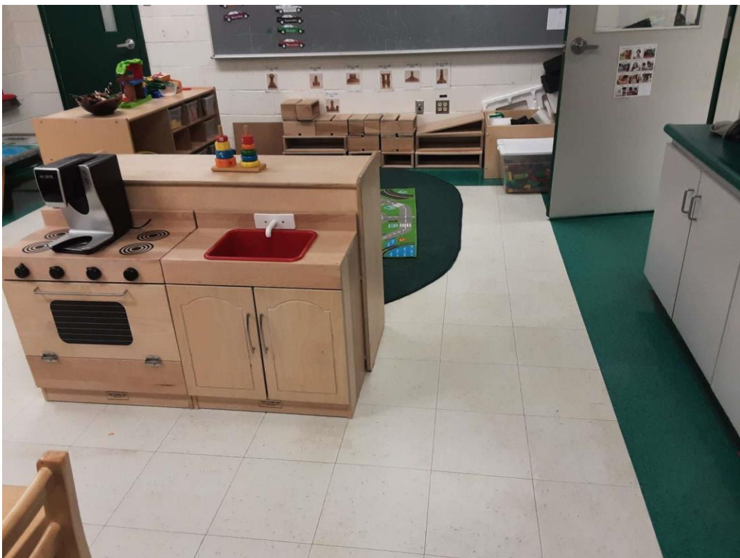
S0012A (Confirmed Asbestos), 12" white with light blue flecks, Floor, All, Vinyl Floor Tile and Mastic, Classroom (Location #: 13)
