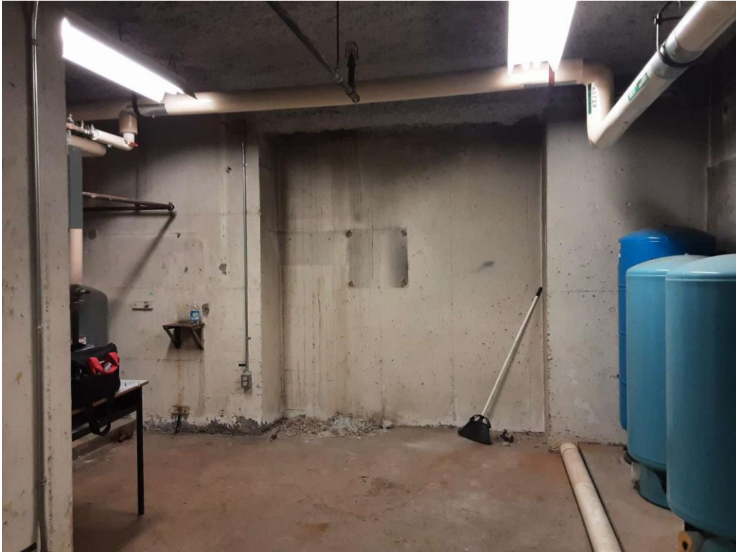
L0001(Lead, Low), White, Wall, Boiler Room (Location #: 1)
