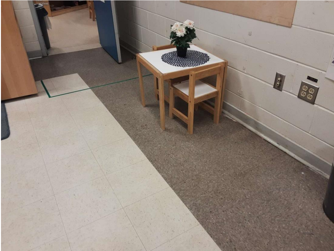
S0011A (Confirmed Asbestos), 12" brown with brown and cream flecks, Floor, All, Vinyl Floor Tile and Mastic, Classroom (Location #: 12)
