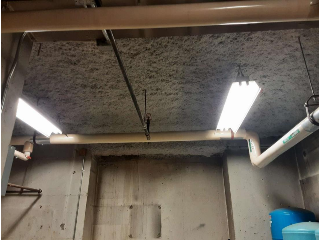
S0001C (None), Grey, Ceiling, All, Fireproofing (Fibrous), Boiler Room (Location #: 1)
