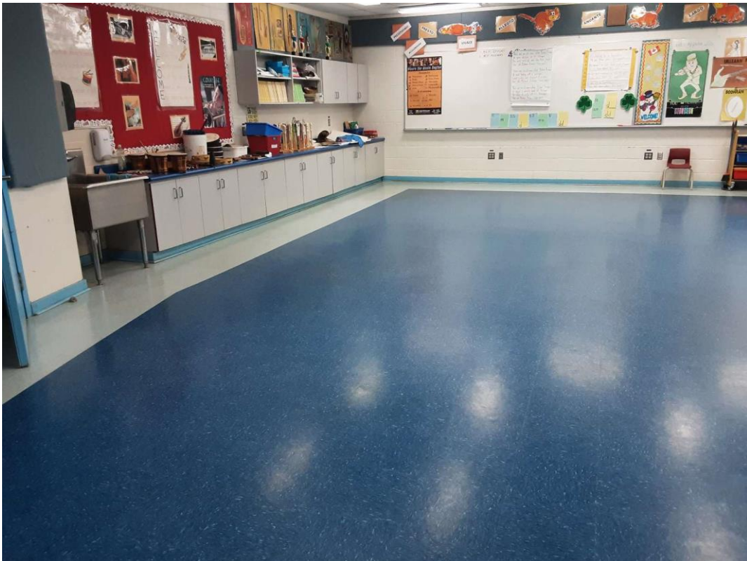
V0000 (None), 12" dark blue with flecks, Floor, All, Vinyl Floor Tile and Mastic, Music Room (Location #: 70) Homogenous installation with other flooring present. No discreet area to sample
