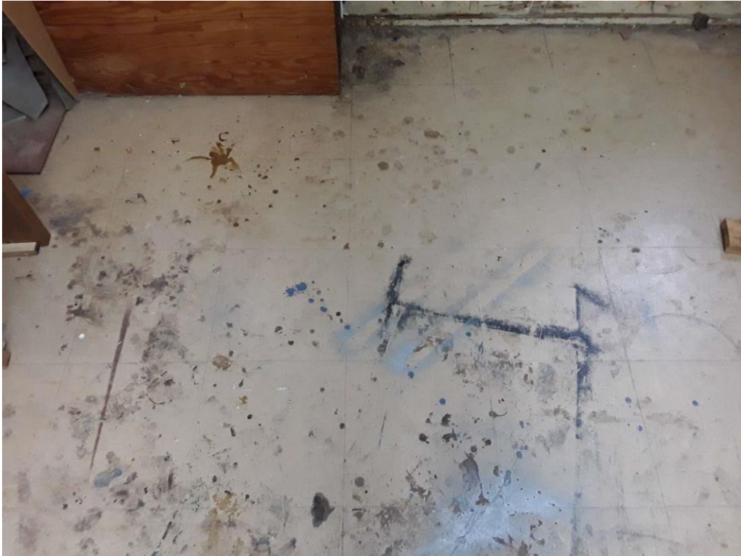
S0018B (Confirmed Asbestos), 12" tan, Floor, Vinyl Floor Tile and Mastic, Lumber Storage (Location #: 35)
