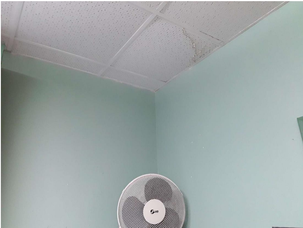
L0010 (Lead, Low), Pale green, Wall, Gym Office (Location #: 29)
