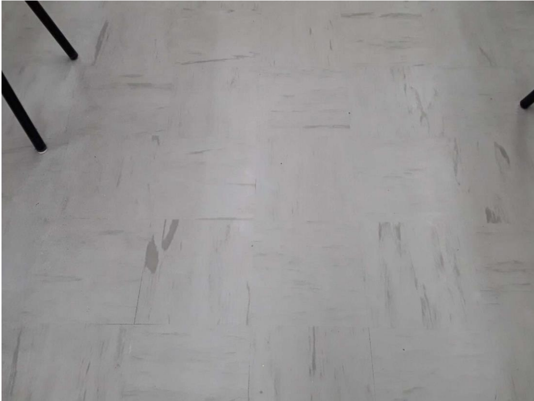
S0008A (Confirmed Asbestos), 12" light green with green streaks, Floor, Vinyl Floor Tile and Mastic, Classroom (Location #: 4)
