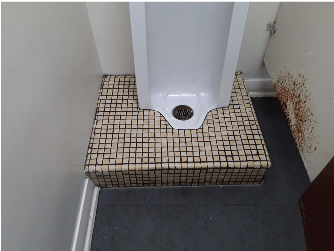
V9500 (Presumed Asbestos), Ceramic tile thinset, Floor, Mortar, Men's Washroom (Location #: 12)
