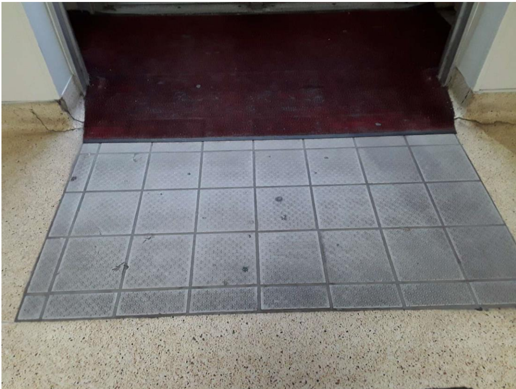
V9500 (Presumed Asbestos), Ceramic tile thinset, Floor, Mortar, Hallway (Location #: 47)
