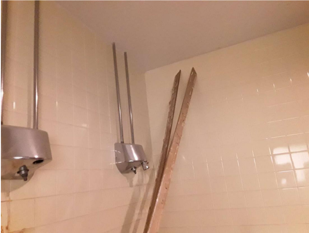
V9500 (Presumed Asbestos), Ceramic tile thinset, Wall, Mortar, Boys Change Room (Location #: 31)
