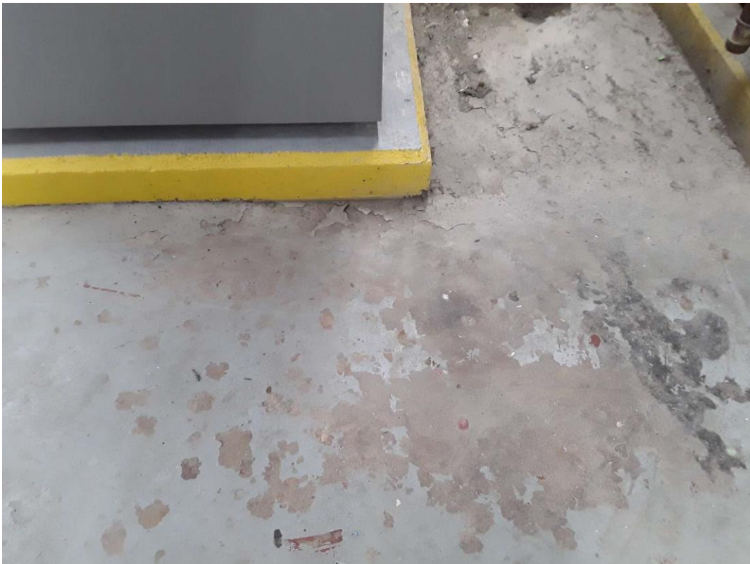
L0003 (Lead, Low), Grey/red, Floor, Boiler Room (Location #: 2)
