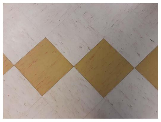
S0027A (Confirmed Asbestos), 12" yellow with red streaks, Floor, All, Vinyl Floor Tile and Mastic, Hallway (Location #. 40)
