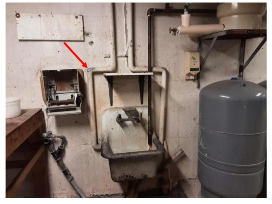
S0002C (Confirmed Asbestos), Piping, Domestic Water (Hot and Cold), Parging Cement, Boiler Room (Location #: 1)
