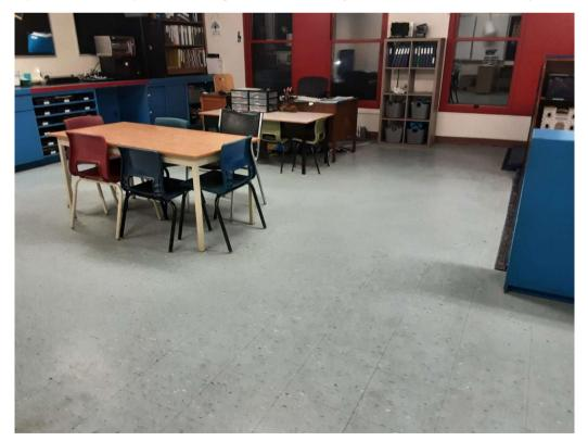
S0018A (Confirmed Asbestos), 12" teal with green and wite flecks, Floor, All, Vinyl Floor Tile and Mastic, Classroom (Location #: 18)
