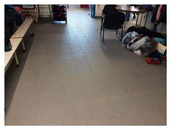
V9500 (Presumed Asbestos), Floor, All, Mortar, Ceramic tile thinset Hallway (Location #: 40)
