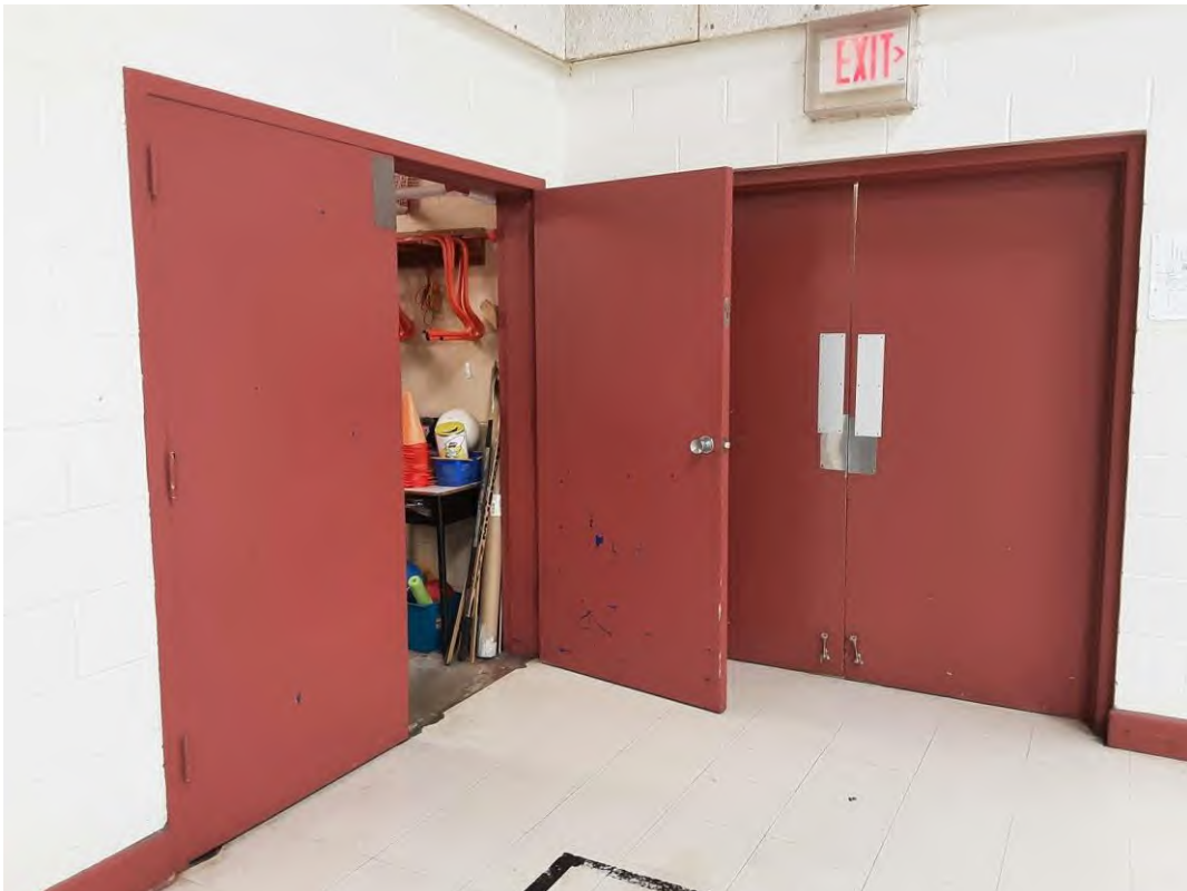
L0007(Lead, High), Red, Door, Gym And Stage (Location #: 28) Blue base, red surface
