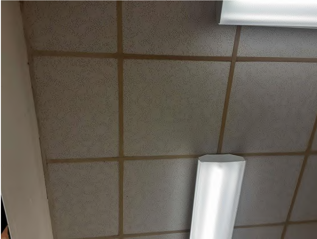
V9500 (Presumed Asbestos), 2'x2' pinhole, Ceiling, ACOUSTIC TILE, Ceiling Tiles (lay-in), Classroom (Location #: 15) Unable to view date stamp or sample due to height.
