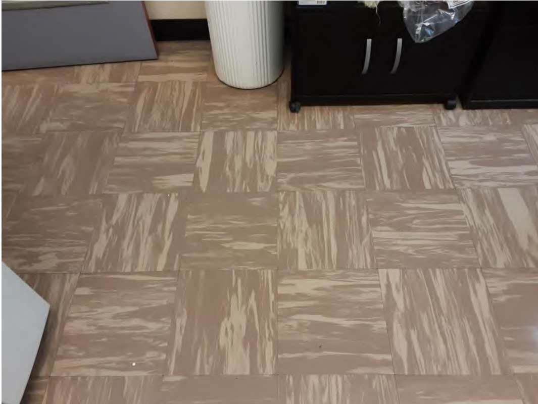
S0008A (Confirmed Asbestos), 12" brown and beige streaked, Floor, All, Vinyl Floor Tile and Mastic, Copier Room (Location #: 3)
