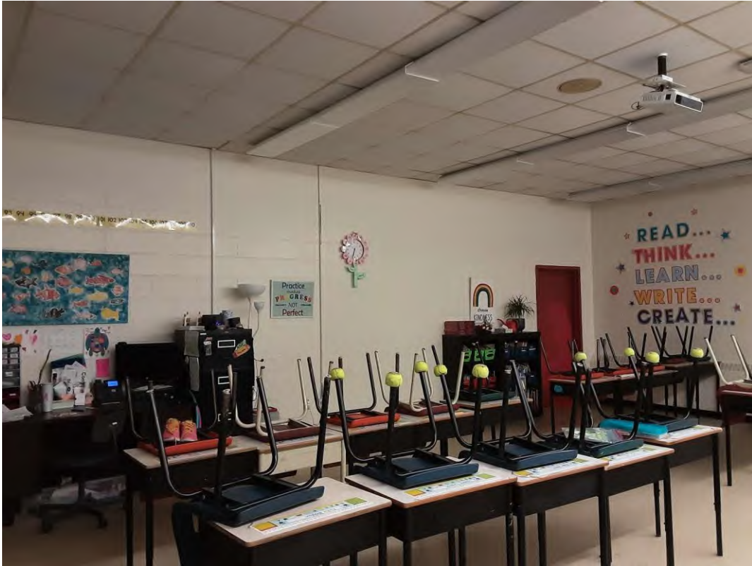
L0004(Lead, Low), Offwhite, Wall, Classroom (Location #: 12)
