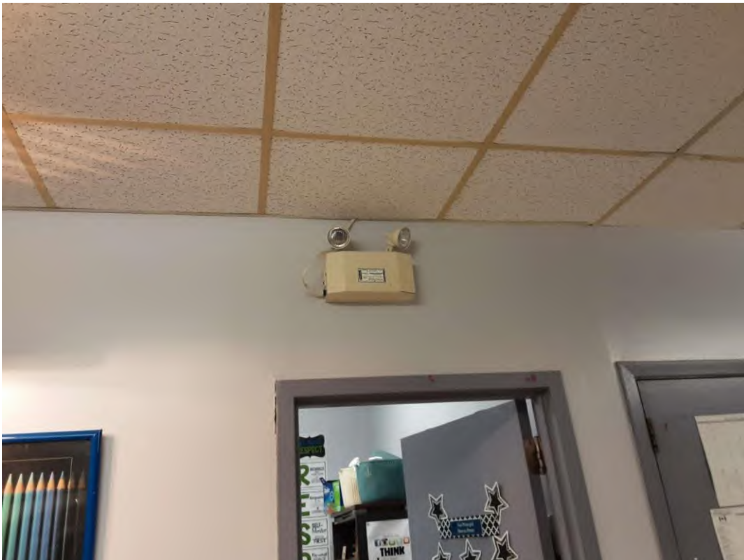
Pb Products, V9500(Presumed), Batteries in Emer. Lights, Administration Office (Location #: 7)
