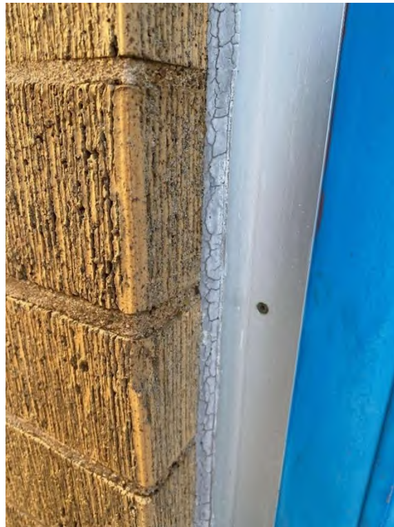
S0030A (Confirmed Asbestos), Grey, Other, Door, Caulking, Exterior (Location #: 76)
