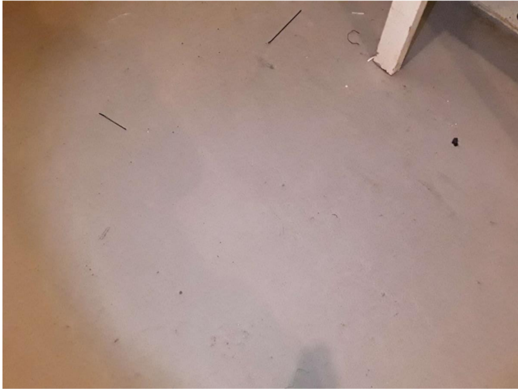
L0005 (Lead, Low), Grey, Floor, Electrical Room (Location #: 7)
