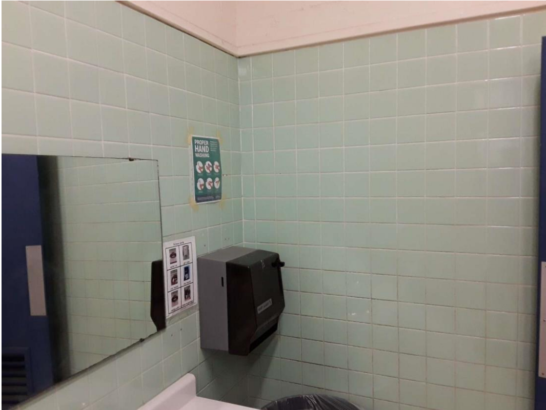
V9500 (Presumed Asbestos), Ceramic tile thinset, Wall, Boys Washroom (Location #: 6)
