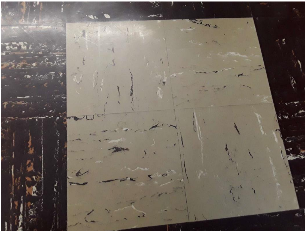
S0040A (Confirmed Asbestos), 9" light brown with white and black streaks, Floor, Vinyl Floor Tile and Mastic, Library (Location #: 35)
