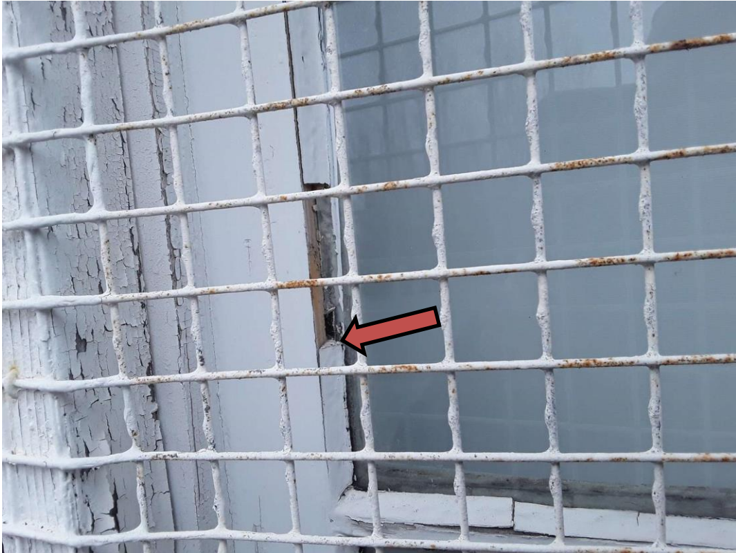
S0025A (Confirmed Asbestos), White, Wall, Window, Caulking (Glazing Putty), Exterior (Location #: 46)
