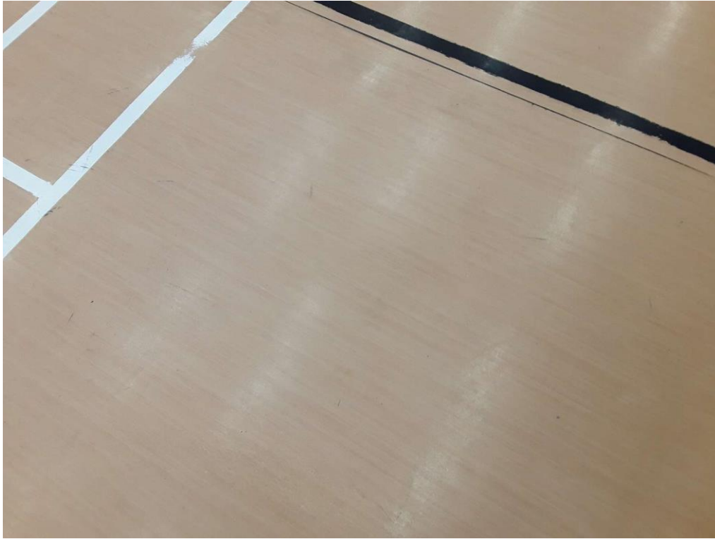
S0020A (Confirmed Asbestos), Light orange, Floor, Vinyl Sheet Flooring (mastic), Gymnasium (Location #: 13)
