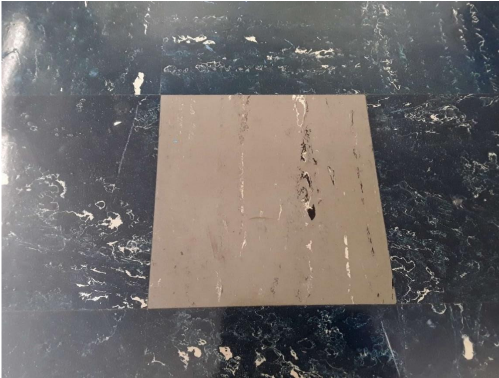
S0035A (Confirmed Asbestos), 9" grey with white and black streaks, Floor, Vinyl Floor Tile and Mastic, Classroom (Location #: 32)
