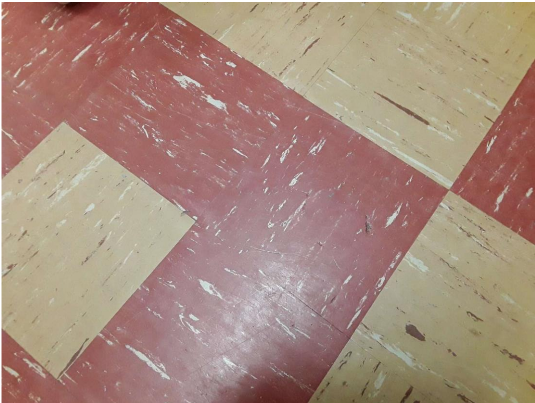
S0005A and S0006A (Confirmed Asbestos), 9" red with white streaks, and 9" tan with red and white streaks, Floor, Vinyl Floor Tile and Mastic, Storage (Location #: 2)
