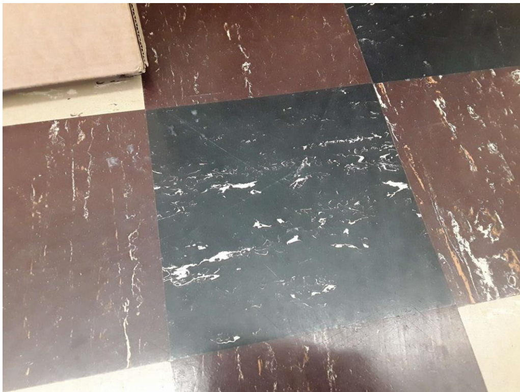
S0042A (Confirmed Asbestos), 9" black with white streaks, Floor, Vinyl Floor Tile and Mastic, Classroom (Location #: 39)
