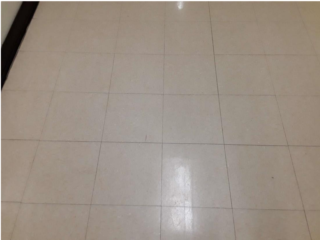
S0032A (Confirmed Asbestos), 12" beige with white and yellow flecks, Floor, Vinyl Floor Tile and Mastic, Hallway and Main Entrance (Location #: 29)
