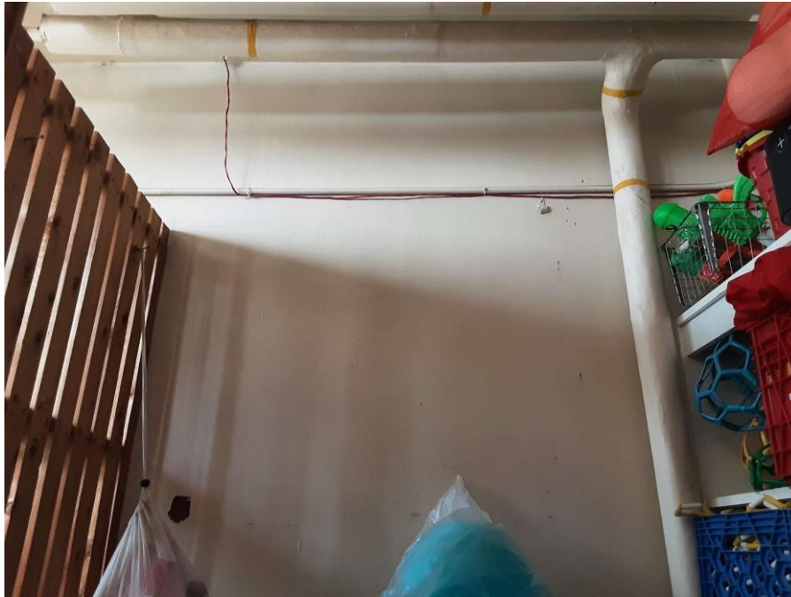
L0002 (Lead (High)), Plaster, Off-white, Sprinkler Room (Location #: 3)
