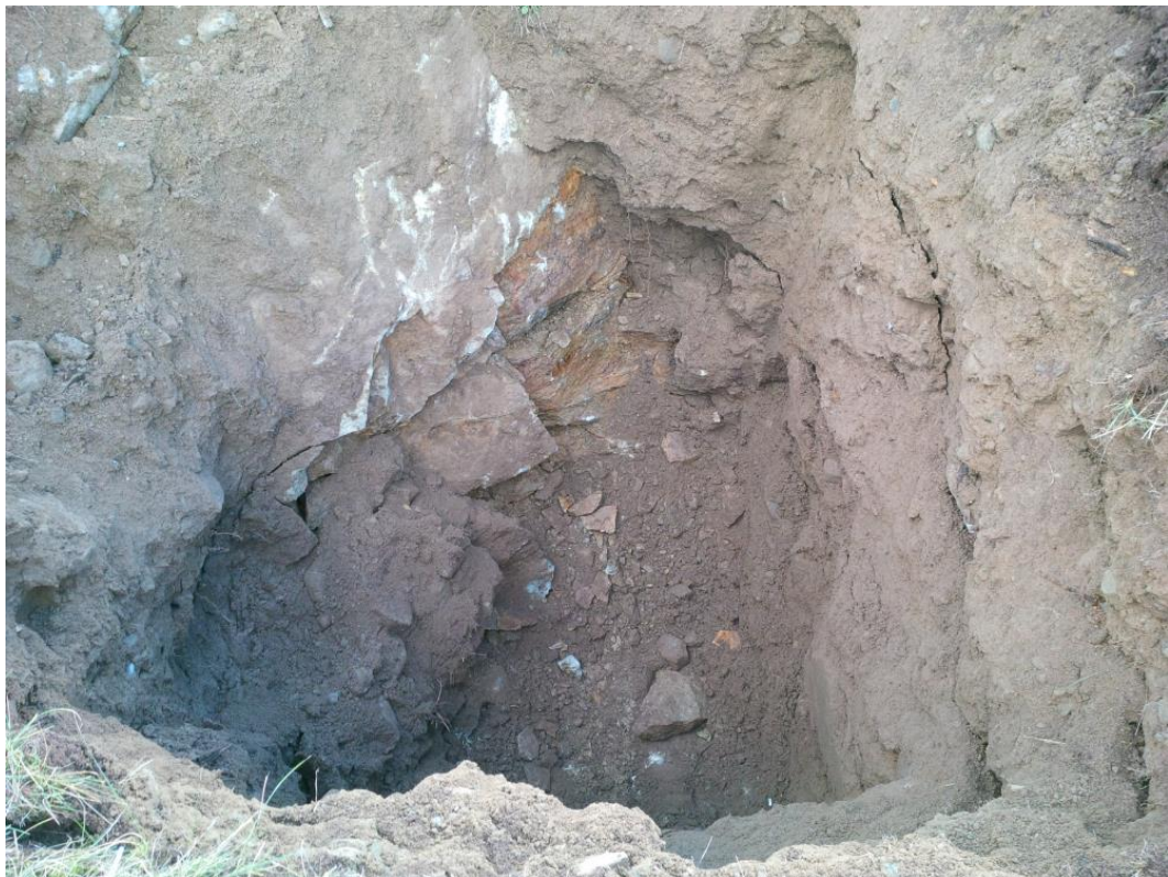
Photograph 8: Test Pit 8. November 27, 2017.
