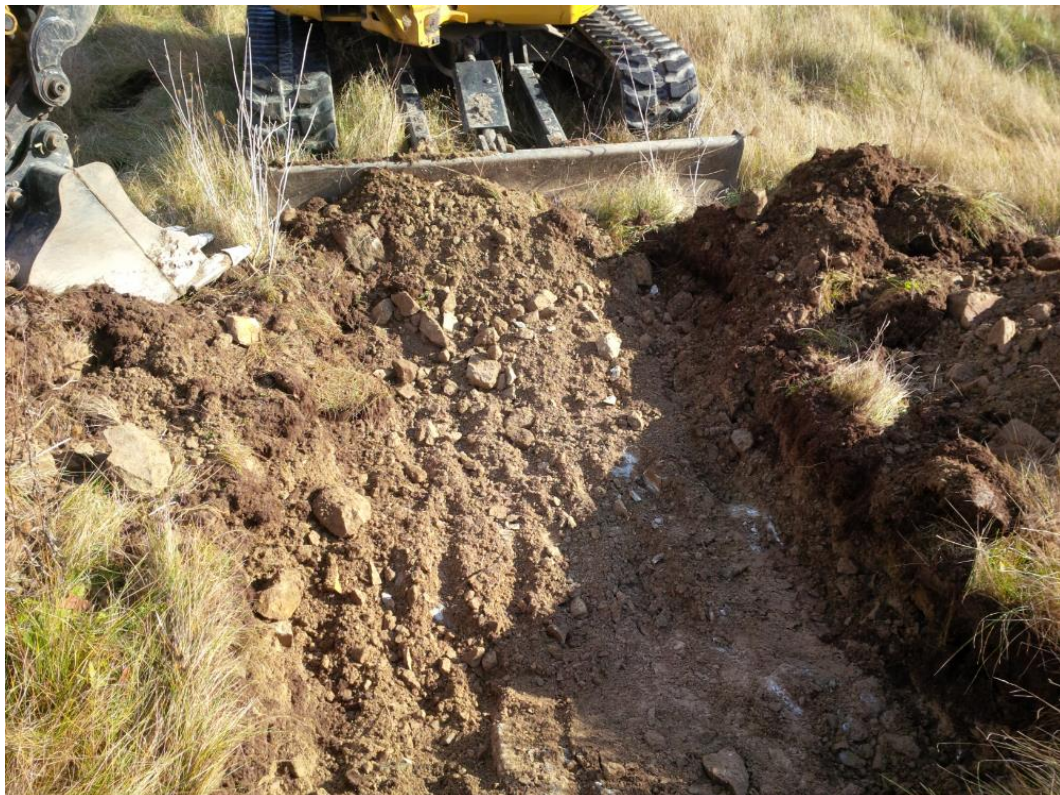
Photograph 6: Test Pit 6. November 27, 2017.
