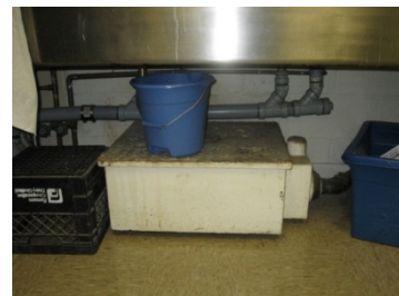
4.3.12 | Pot Sink grease interceptor
