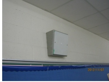
3.7.2 | Typical P/A System Speaker
