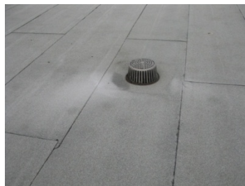
4.2.2 | Roof drain with cast dome
