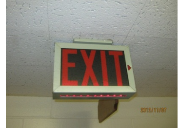
3.3.6 | Typical exit sign retrofitted with LEDs
