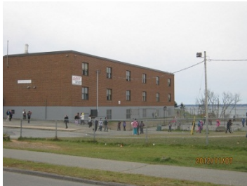
3.1.1 | Overhead Electrical Service
