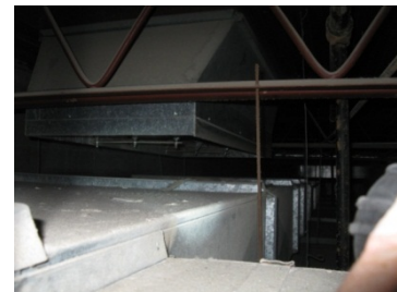
4.6.3 | Return air relief hood from R/A plenum
