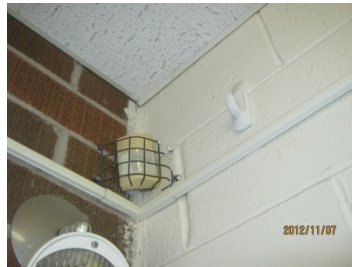
3.8.2 | Wall Motion Sensor
