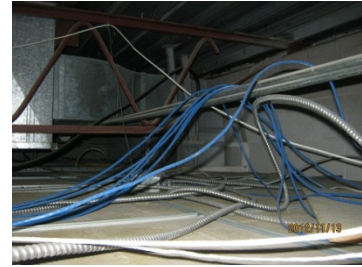
3.5.6 | Communications wiring retrofit in ceiling space
