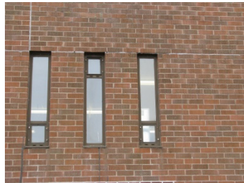
1.3.2 | Overall view of typical cafeteria window configuration
