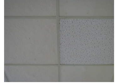
2.2.6 | Replacement ceiling tiles
