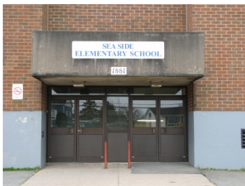
1.5.1 | Precast soffit at main entrance
