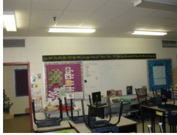
4.6.5 | Typical sidewall supply and return grilles
