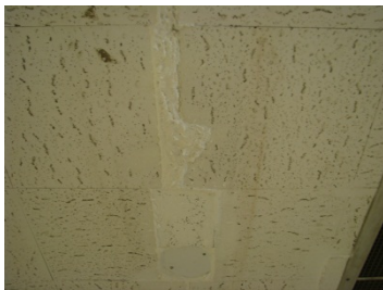
2.2.1 | 12"x12" tile reattached with foam adhesive
