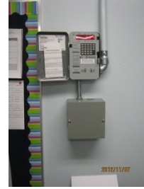
3.7.3 | Class Dismissal Time Clock
