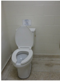
4.3.1 | Typical Barrier free Water Closet
