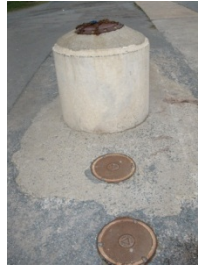
4.4.8 | Underground oil tank
