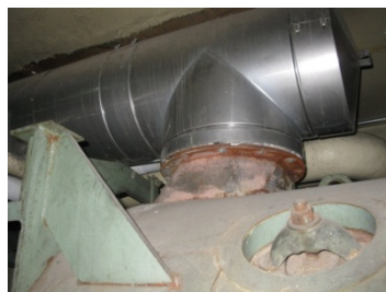
4.4.2 | Boiler breeching replaced
