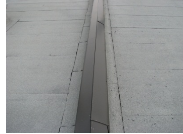
1.1.6 | Roof expansion joint
