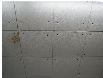
2.2.2 | 12"x12" ceiling reattached with drywall screws
