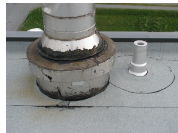
1.1.3 | Chimney and plumbing vent flashings
