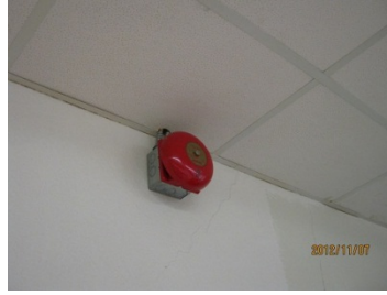
3.4.2 | Typical fire alarm bell
