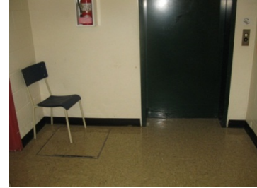
4.3.15 | Elevator sump pit by Boiler Room
