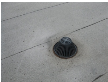
4.2.1 | Roof drain with plastic dome
