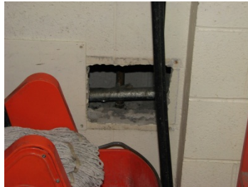
2.3.5 | Penetration through wall in Janitor's Closet 324
