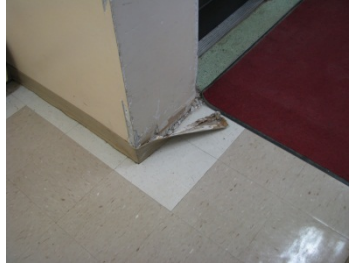
2.1.2 | VCT-1 at Main Entrance elevator alcove.
