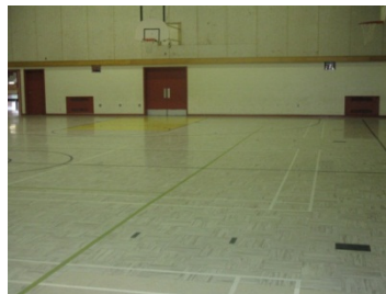
4.5.5 | Gym Cabinet Heater
