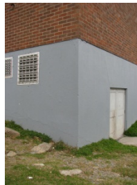
1.2.5 | Exterior foundation wall at SW corner
