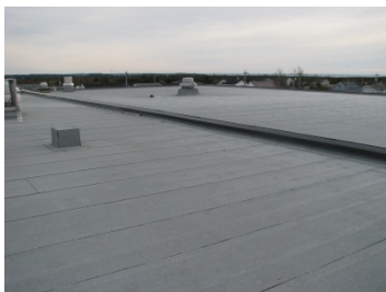
1.1.1 | Existing (reroofed) roof
