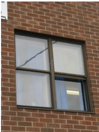
1.3.1 | Overall view of typical window configuration
