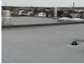
1.1.5 | One of the four roof drains
