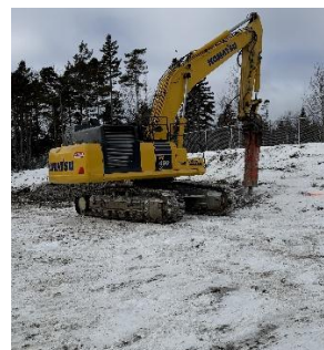
Rock breaking for sanitary and storm lines
