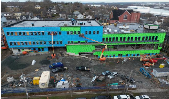
Building Structure - end-November 2024
