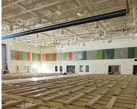
Gymnasium floor started mid-Nov
